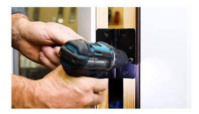
Completely fill with sealant any hinge screw holes that penetrate the frame into the RO (outswing).
