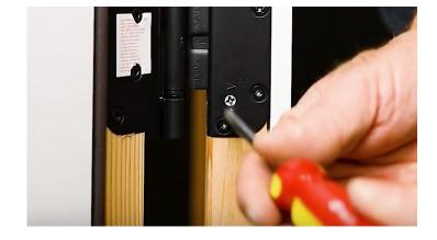
The rest of the hinges will have a screw marked "H" for horizontal which will move the panel left to right. Having a second person hold the door panel at the opposite edge can make this process easier.
