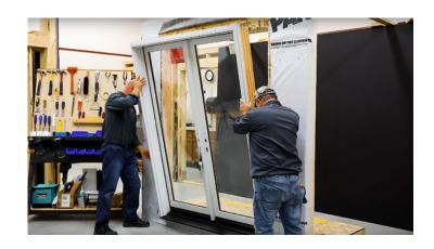
Tilt the door up and push the top of frame into place.
