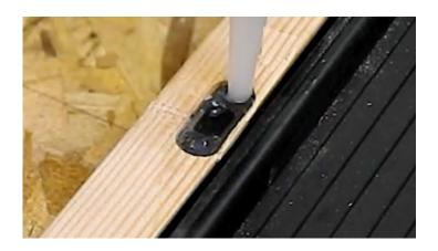
Place the plate, then insert long screws from the hardware package into the holes.
