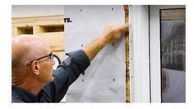
Ensure that screws go in straight and perpendicular and not angled, to avoid creating a bow in the jamb, creating wide cavities in between frame and rough opening.
