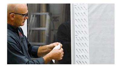
Apply slices of window/door flashing over the diagonal cuts made in the WRB. Ensure that the entire cut is covered.
