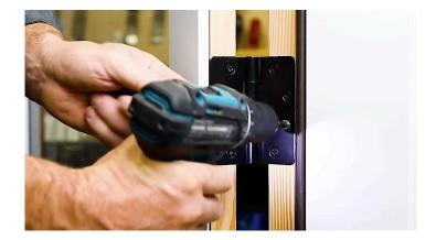
Completely fill with sealant any hinge screw holes that penetrate the frame into the RO (outswing).
