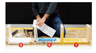
All Sill Pans should be sloped to outside with a minimum 1/2" interior upturn leg or dam and 2" exterior down turn leg. Upturn frame at jamb end should be 6".
