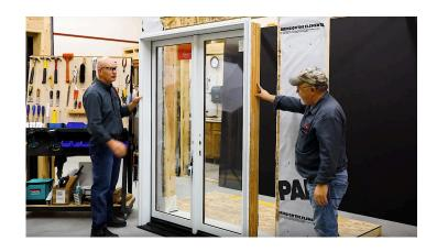
Set the door from the exterior into the rough opening, starting with the bottom edge, on the sill pan. The jamb legs should be sitting on the sill shims on each side.
