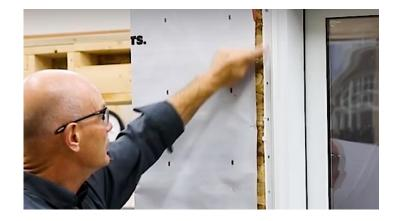
Ensure that screws go in straight and perpendicular and not angled, to avoid creating a bow in the jamb, creating wide cavities in between frame and rough opening.
