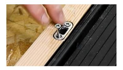
drill longer pilot holes into the sill pan, then fill holes completely with clear silicone sealant.
