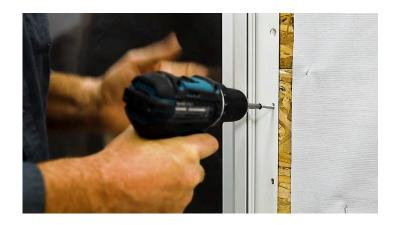
Over and under tightening hinge anchor screws will affect the door reveals.
