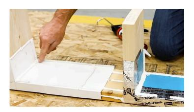
On the rigid sill apply a sealant bead on top of the sill pan flashing along the exterior of the rough opening, leaving a 2" void approximately 2" from either end. This will allow a drainage path for incidental moisture.
