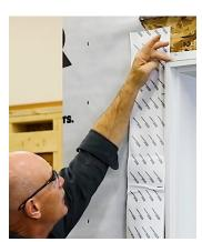
Apply flashing to the exterior wall along the edge of the door frame over the flange, extending approximately 4" above the top of the frame.
