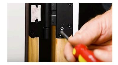
The top hinge will have a screw marked "H" for horizontal which will move the panel left to right. Having a second person hold the door panel at the opposite edge can make this process easier.
