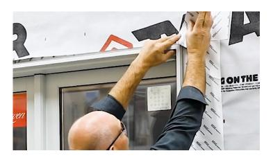
Note: If a rigid head flashing/ drip edge hasn't been factory installed, ensure an appropriate one is installed correctly.
