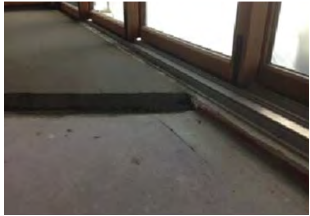
Filling in Concrete Base
