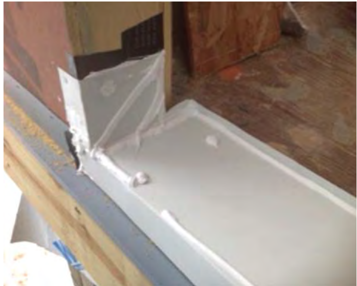
Rigid Sill Pan Installation
