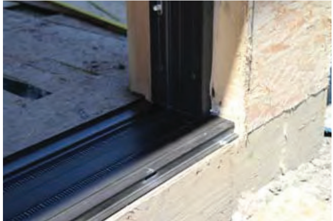
Raised Track Without Nosing Piece
