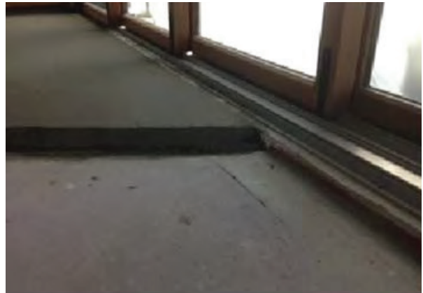
Filling in Concrete Base
