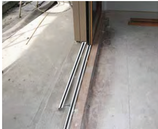
Filling in Concrete Base
