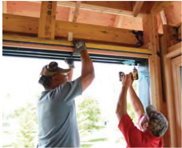
Head Track Installation
