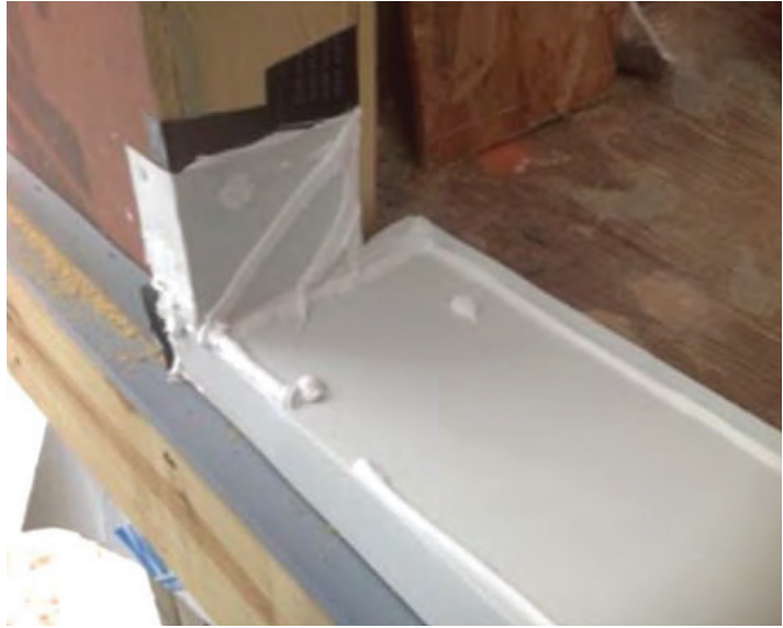
Rigid Sill Pan Installation
