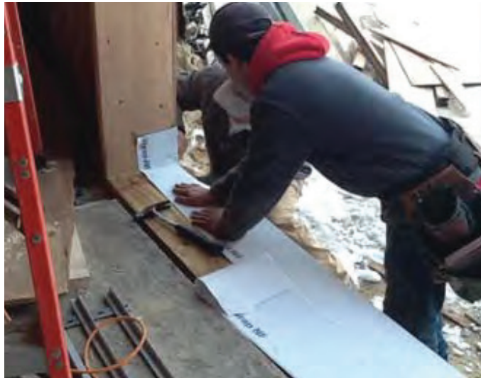
Flexible Sill Pan Installation
