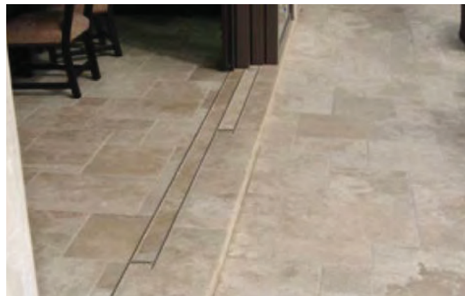
Finished floor of a flush track assembly
