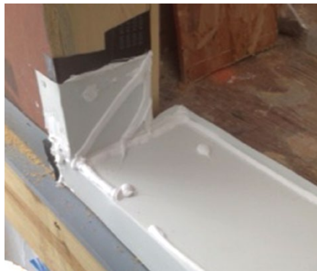
Rigid Sill Pan Installation
