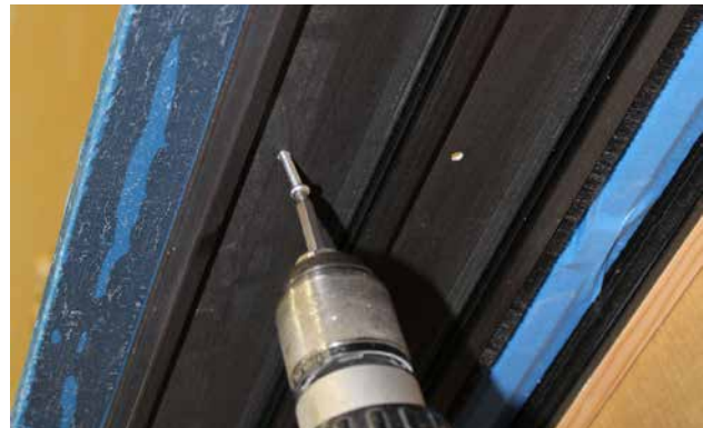
Head flashing with appropriate fasteners. Seal over fasteners with Sealant.
