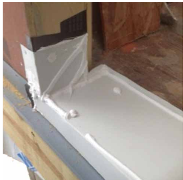
Rigid Sill Pan Installation
