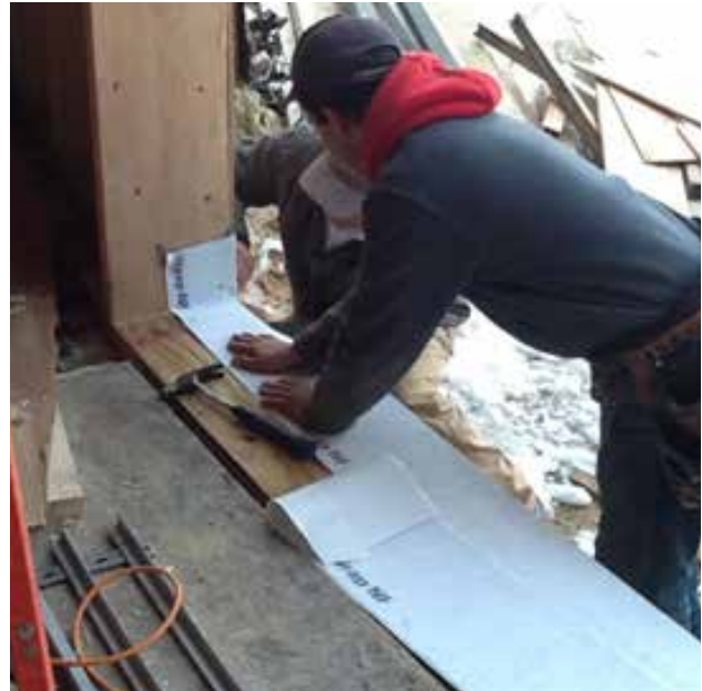
Flexible Sill Pan Installation
