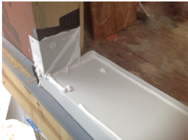
Rigid Sill Pan Installation
