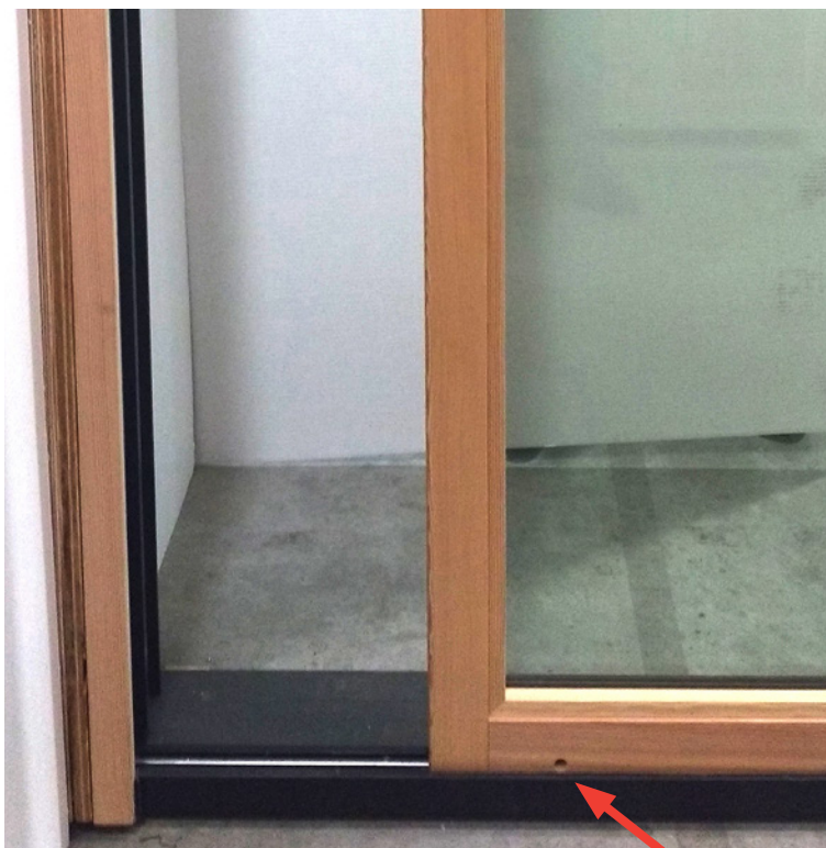
WHEEL ADJUSTMENT ACCESS HOLES
