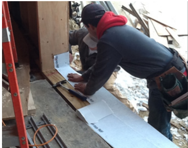
Flexible Sill Pan Installation
