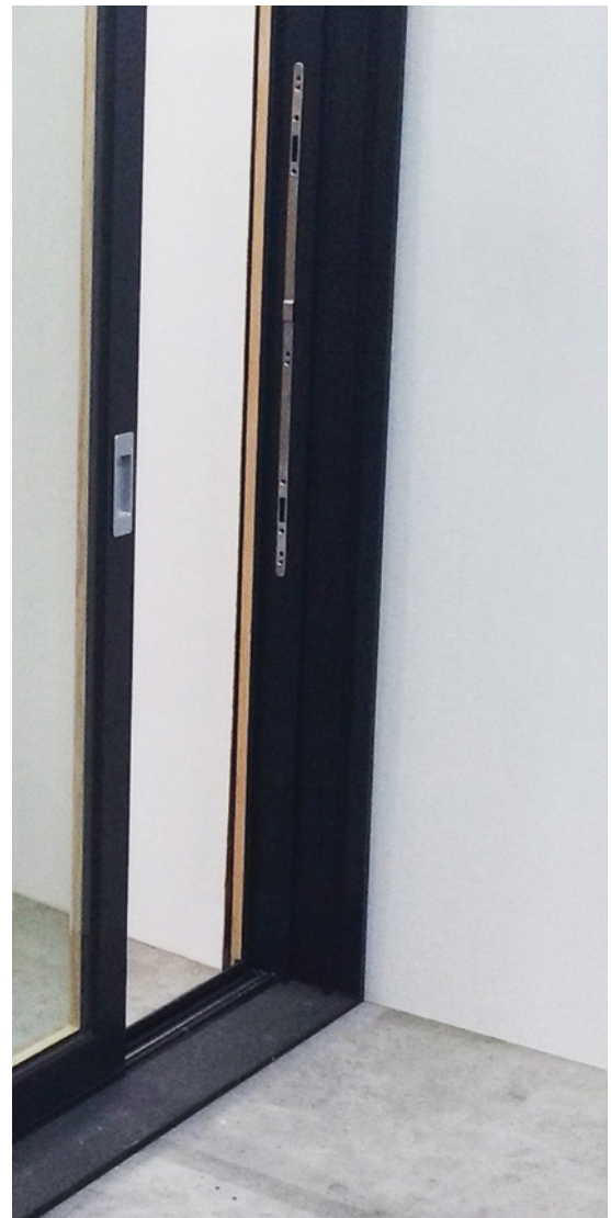
FINAL DOOR ASSEMBLY (PANEL INSTALLED FOR REFERENCE ONLY)
