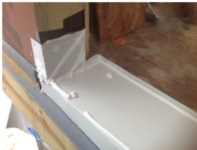
Rigid Sill Pan Installation
