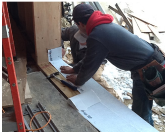
Flexible Sill Pan Installation
