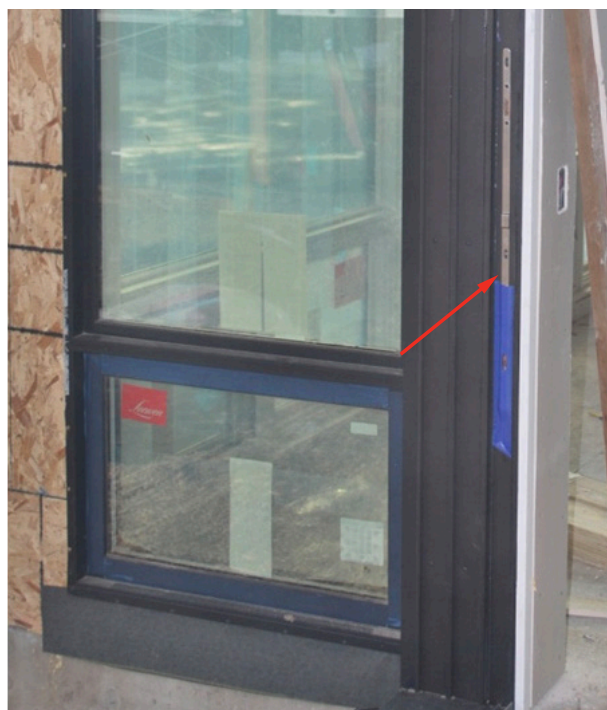
Interior track with spike plate
