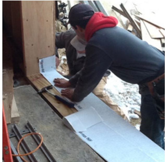
Flexible Sill Pan Installation
