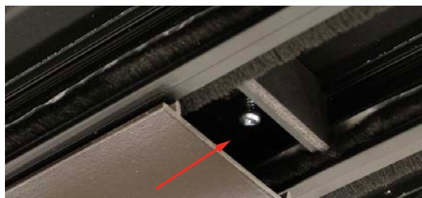
Head track cover will be installed after stops, shown for visual location only
