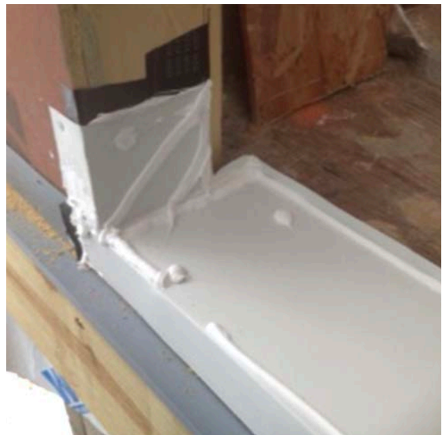
Rigid Sill Pan Installation
