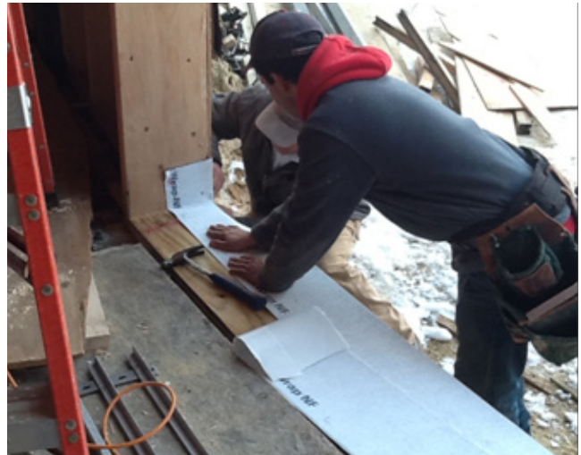
Flexible Sill Pan Installation
