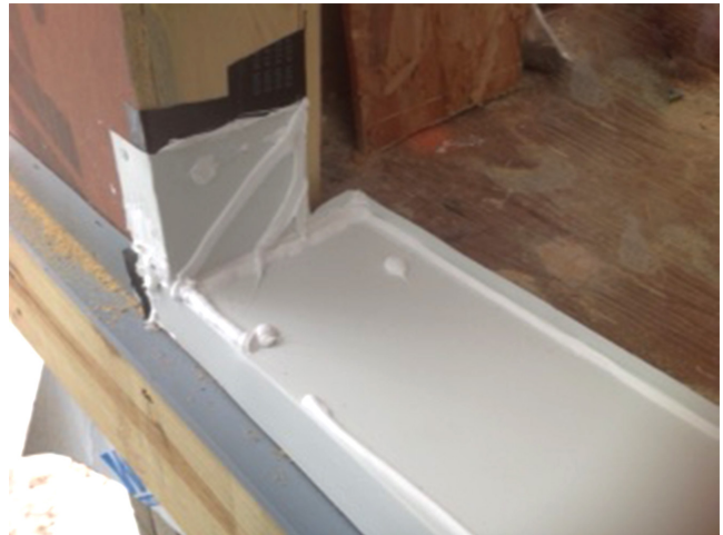
Rigid Sill Pan Installation
