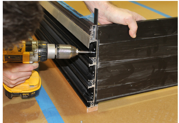
Jamb Assembly screws
