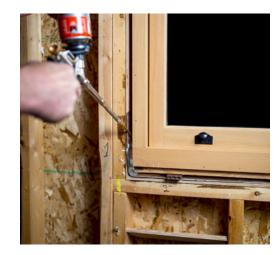
Note: After the foam has set you may fill the entire rough opening cavity with closed-cell foam or fiber glass insulation.
