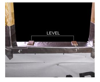
Note: In a future step, the foam being applied under the window needs to be a continuous seal at the sill.
