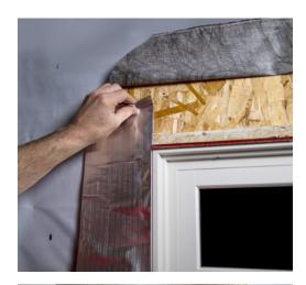
Note: If a rigid head flashing/drip edge hasn't been factory installed, ensure an appropriate one is installed correctly.
