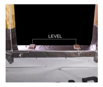
Note: In a future step, the foam being applied under the window needs to be a continuous seal at the sill.
