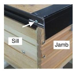
m. Attach foam block (#49808BLK) onto lock side jamb.Note: Step m. applies to 2 wide or 3 wide units only.
