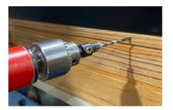
e. Secure fixed panel in frame with #8 x 2 <sup>1</sup>/<sub>2</sub>" screws (#316139) in each hole.
