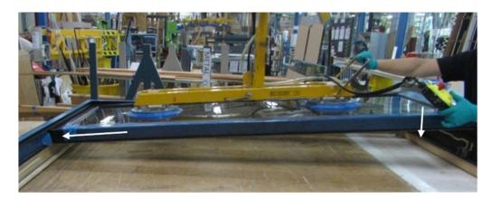
c. Ensure panel is tight to jamb and tight to frame cladding lip, clamp as required.
