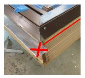
f. Secure head flange to head ensuring ends lap over side flange ends, compressing the sealant applied in step e.
