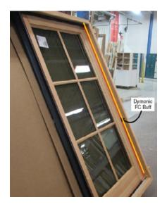
b. Fasten interior moulding to jamb with 1 <sup>1</sup>/<sub>4</sub>" light finishing or pin nails, spaced 150mm (6") apart. (Not included).
