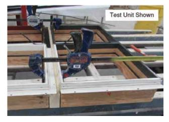
3. Apply 10 mm continuous bead of Dymonic FC Buff (#297837)) along entire length of mull and mitre joint. (orange line shown)
