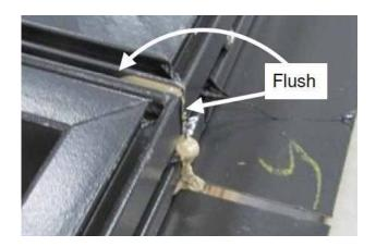
6. If casing is required or more units are required to be part of combination (e.g. 3 wide); apply temporary pieces of mull cover or clamps to hold units together.
