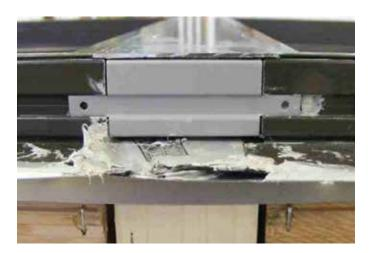
2. Secure mullion joint cover with two 6 X  $^{1/2}$  screws (#305632).
