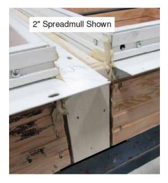
6. For frame side(s) with flange, apply #6 x 1/2 SS PH SQ (#320456) through each hole on the flange into spread mull.
