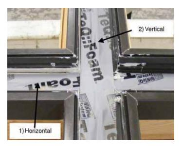
**Note:** Vertical tape must overlap horizontal tape. This applies regardless of spreadmull orientation. 3. Apply a continuous bead of Dymonic FC Buff (#297837) along entire length of mull covering tape and frame joint on both sides of mull.
