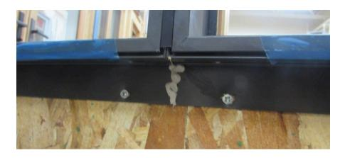
10. Flatten all sealant beads as shown.
