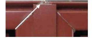
4. Use a rubber mallet and a vinyl block or wood block to snap mullion cover into kerf as shown.
