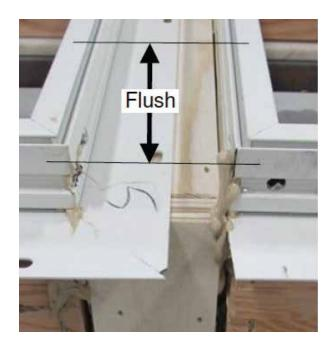
**Note:** Ensure spread mull and both units are flush on ends and interior face.
