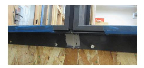
11. Apply flange tape over face side of each bottom flange joint.
