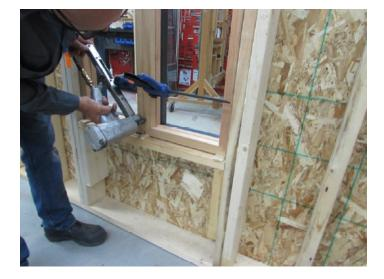
9. Seal gap at each flange joint with Bostik Pro MS50 (#49819).
