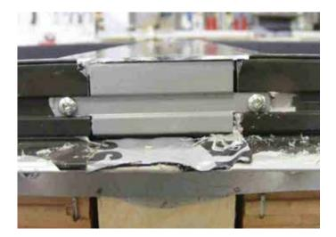
Apply a 5mm bead of Bostik Pro MS50 (#49819) on nailing flange, in a box pattern as shown, and along the flange joint on both interior and exterior sides.
