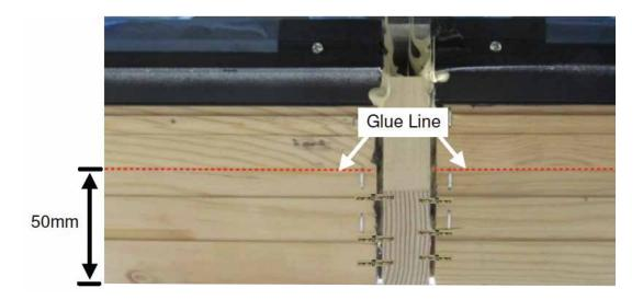
1. For frame side(s) with flange, apply  $#6 \times 1/2$  SS PH SQ (#320456) through each hole on the flange into spread mull.
