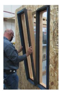
5. Clamp units together, as required, from interior and exterior.
