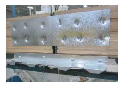
4. Crimp all 4 tabs minimum 3 times each to ensure the mullion flange plate is completely flush with nail fin.
